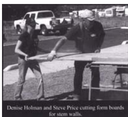
Denise Holman and Steve Price cutting form boards for stem walls.
